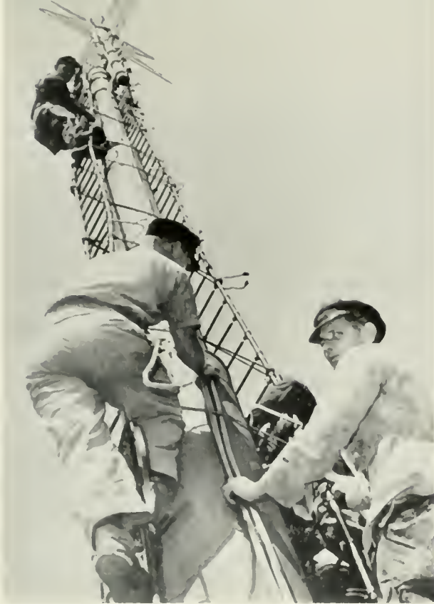
This bat-wing transmitting antenna erected atop West Berlin's City Hall gave German residents their first glimpse of American television.
