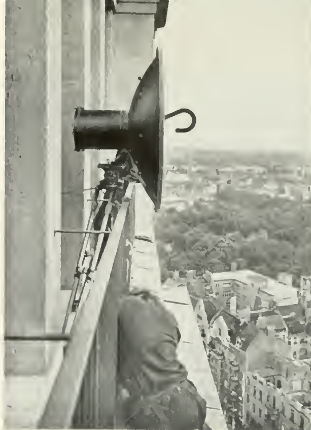
One of the two microwave relay units used in the Berlin telecasts was mounted on the side of the City Hall tower, one of the highest points in the area.
